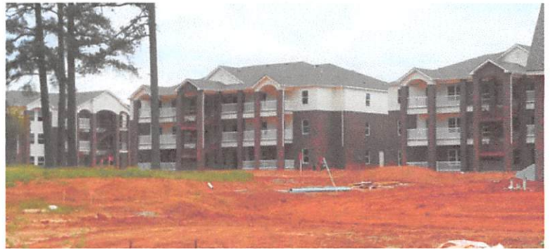
The Longhills project is adding 612 multifamily units north of I-30 in Benton.
